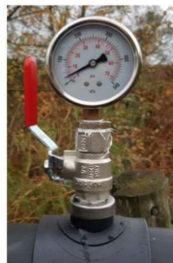
|Pressure gauge installed in a tapped hole - Gauge installed in a reducing bush
