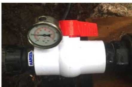
|Pressure gauge installed in a tapped hole - Gauge installed in a reducing bush
